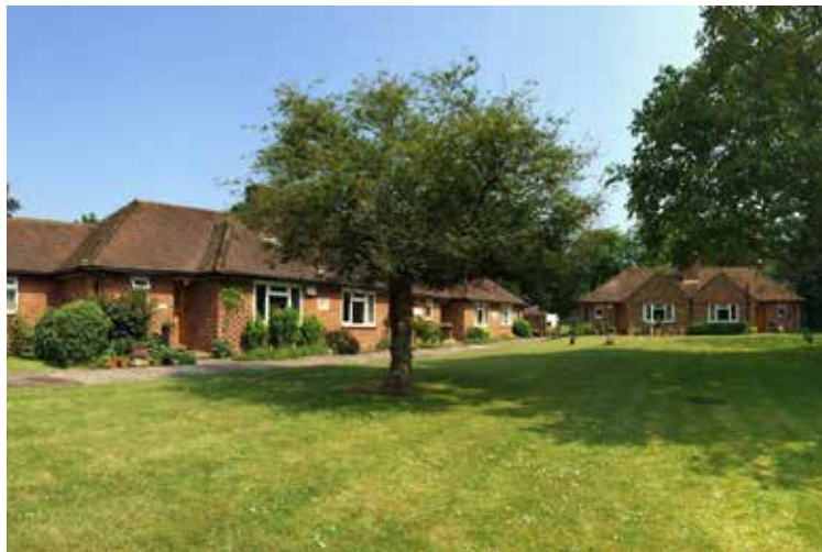
Hedger's Almshouses, Wykeham Road in Merrow.
